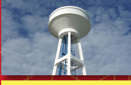
Overhead water tanks
